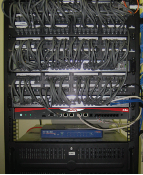
Transonic Combustion's Allworx 24x system on an equipment rack at their Camarillo location.
